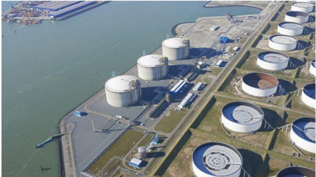
Figuur 3: Gate terminal in Rotterdam, © Aeroview, overgenomen van [8]
