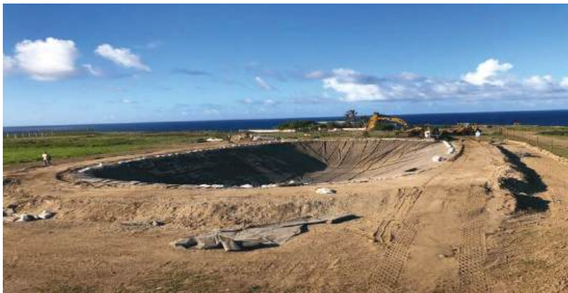
Figure 4.4 Water retention pond under construction near the St. Eustatius solar park. Source: St. Eustatius government
