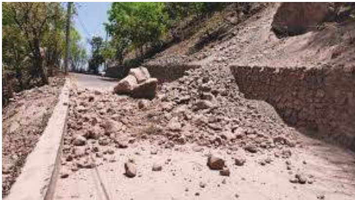
Figure 3.7 Landslide striking a major road on Saba
