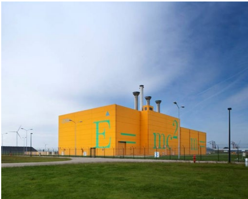
Figure 5.4: HABOG before current extension.
