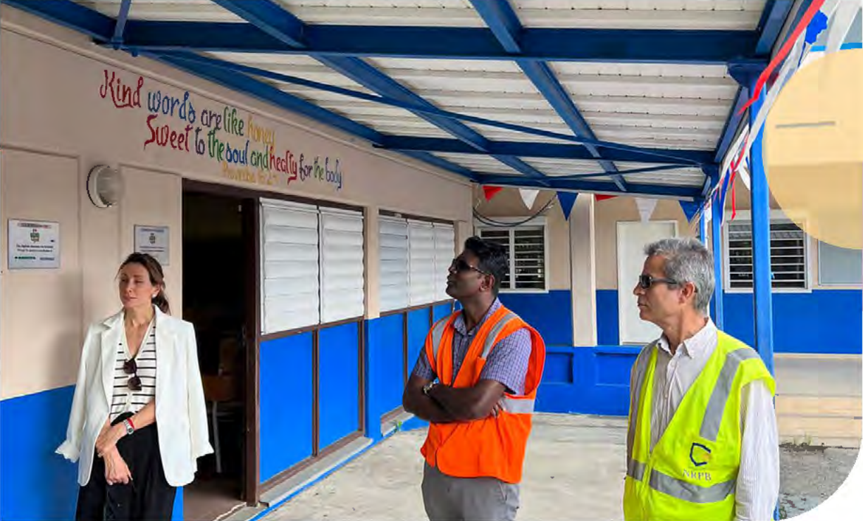
Reviewing progress at Helmich Snijders Hillside Christian School during World Bank implementation support mission in May, 2024.
