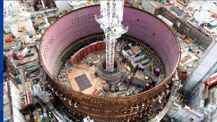
Fig 5: Hinkley Point C construction of the second reactor ( link )
