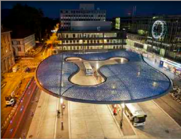
4. Aarau Bus Station canopy
