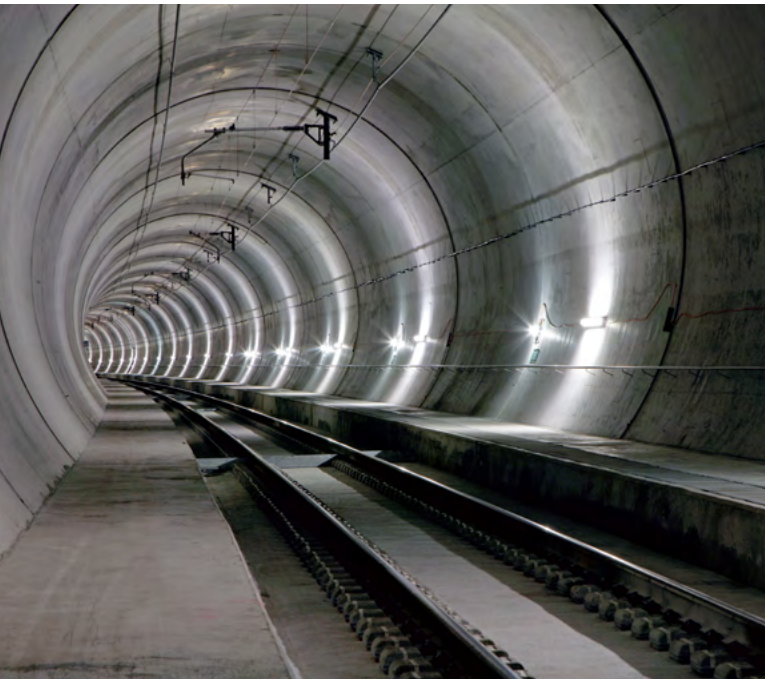
Inside the Lötschberg base tunnel.
